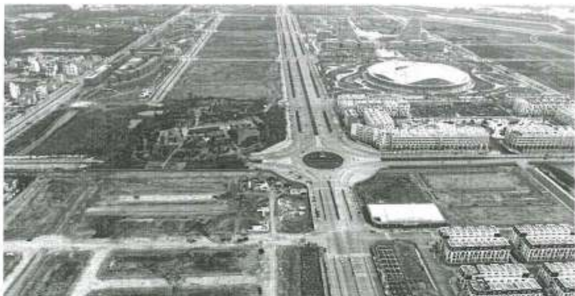
A corner of the project under construction looks towards the new administrative center of Hai Phong City in April 2025.
