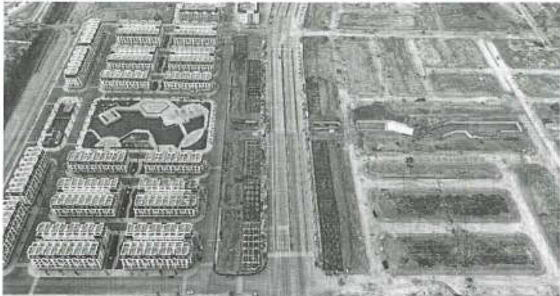
The project is leveling the ground and implementing the construction of internal infrastructure, building a number of adjacent housing areas
