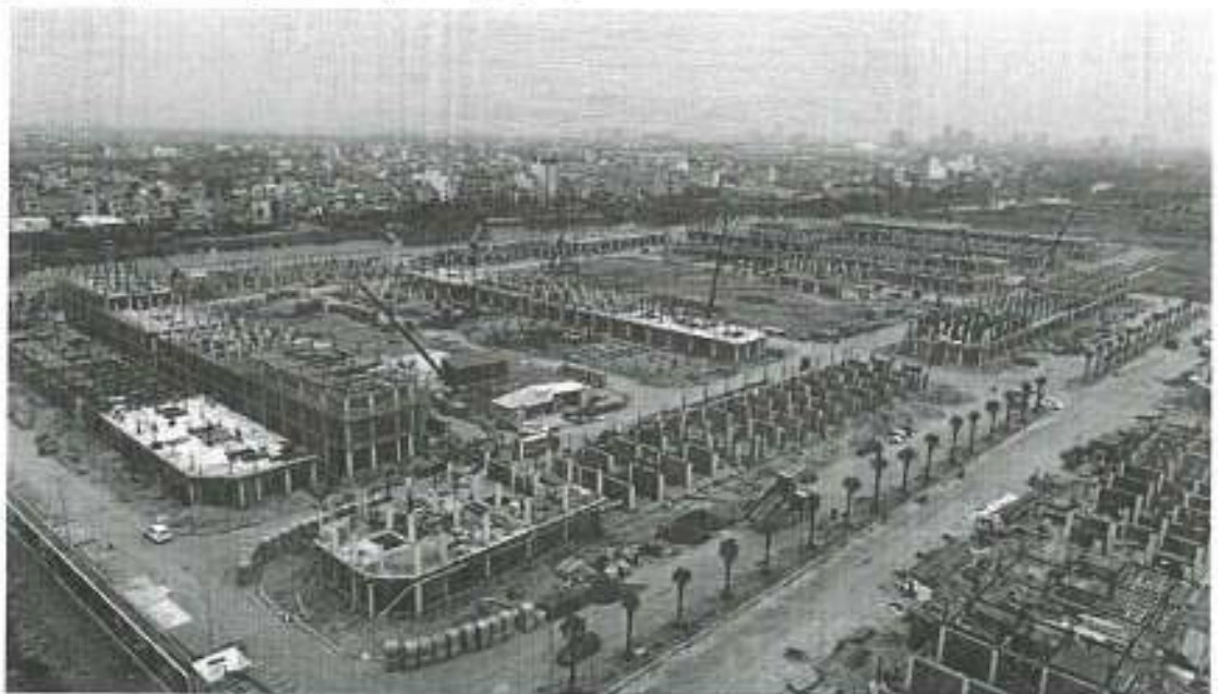
Close-up of the construction progress of house blocks in April 2025
