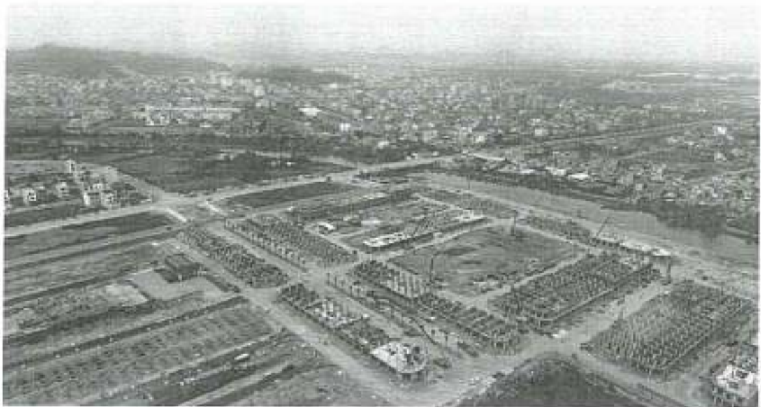
The project is implementing construction simultaneously, many housing items are gradually forming at the beginning of April 2025
